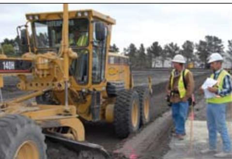
GCC's contributions to the Cader Corporate Center project include grading and clearing the 15-acre site, and its 200,000 square feet of building pads. GCC is stabilizing the soil with lime treatment; installing underground utilities (sewer, water, and storm drainage); providing the concrete flat work (curb and gutter) and drop inlets; and AC paving.
